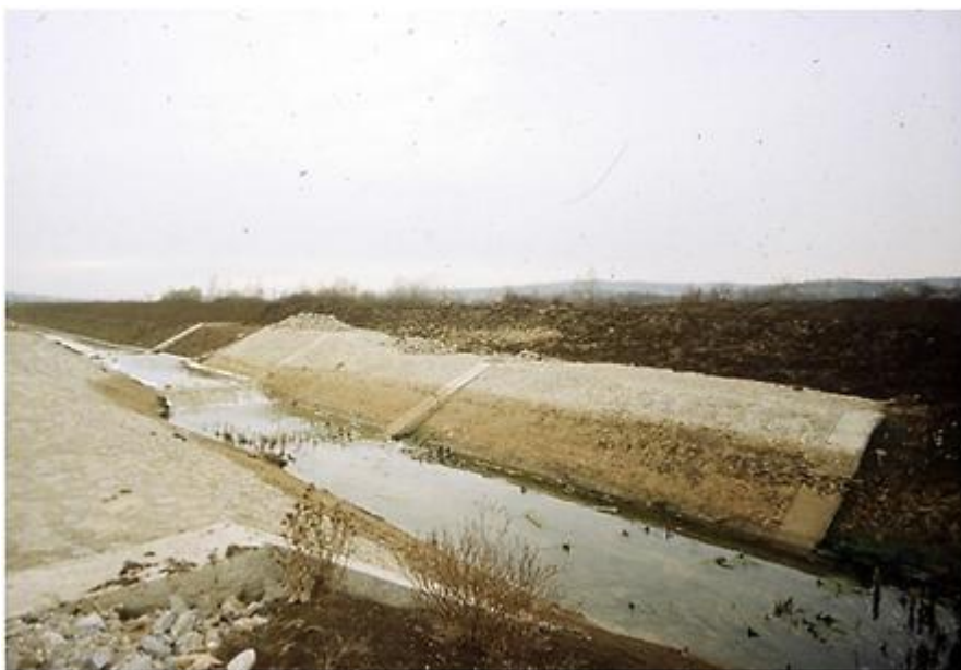
Figure 3. Regulation of the River Ralja with the local enforcement of flow profile (Photo: V. Djekovic, 2012)
